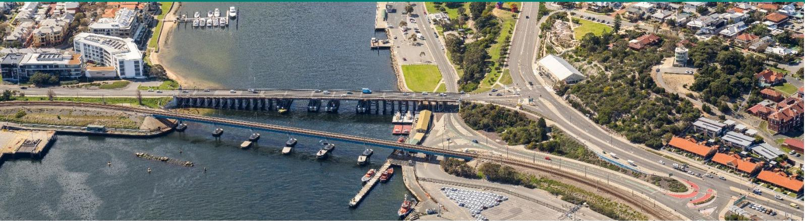
The Fremantle Traffic Bridge houses telecommunications, gas and water services that need to be removed from the deteriorating bridge.
